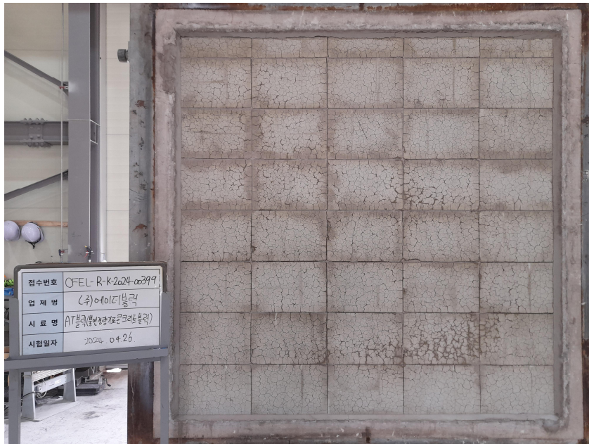
< Exposed face – after test >
